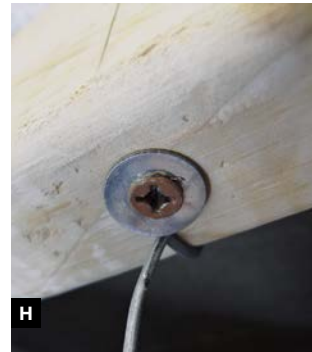
upright. Fig. E: Cross section showing how the shelf is attached to the wall. Figs. F–H: A wood rack was made from pine 2×4s with 2½" wheels attached. Galvanized wire separators are secured with screws and washers.
